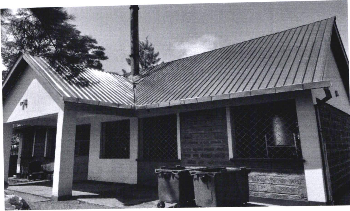
Fig1: Front; Renovated Incinerator housing and the machine
