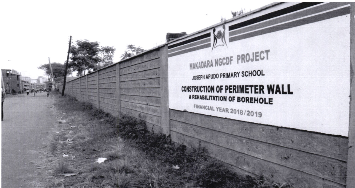
Perimeter Wall at Joseph Apudo Primary School and Rehabilitated Borehole.
