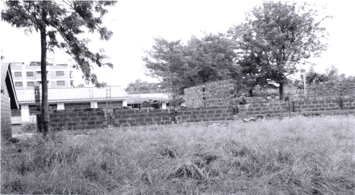
Ongoing Proposed Construction of 4 classrooms at St Anne's Girls Secondary School
