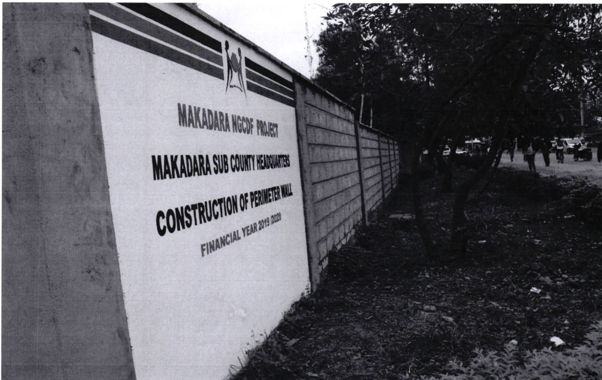
Perimeter Wall at Makadara Sub County Headquarters
