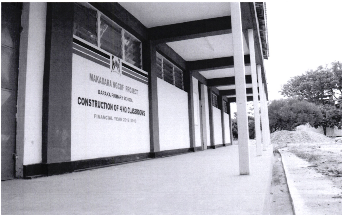
4 no of new classroom at Baraka Primary School.
