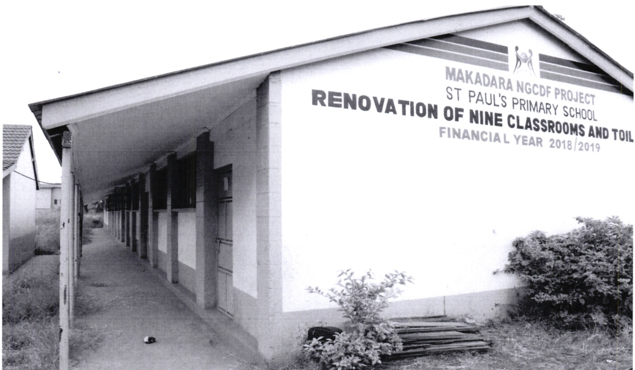
Rehabilitation of Classroom at St Paul Primary School
