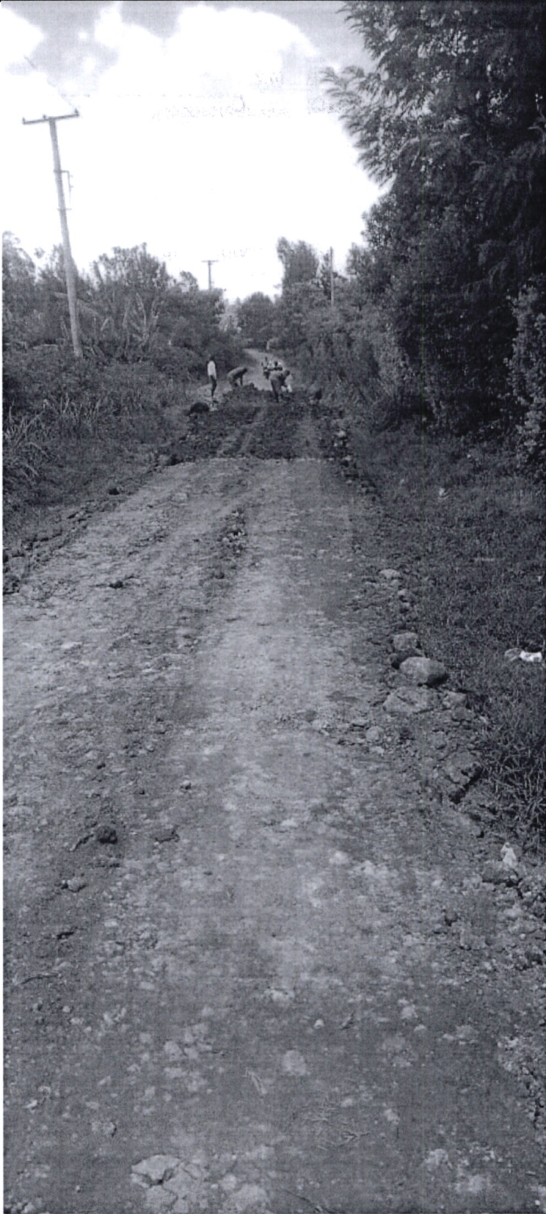
Access road repairs in Embu Zone
