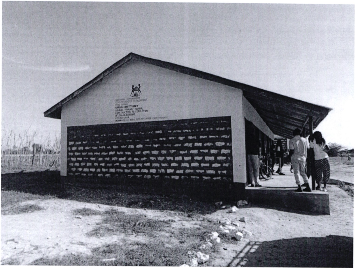
Ushindi Primary school -construction of 2 no. of classrooms
