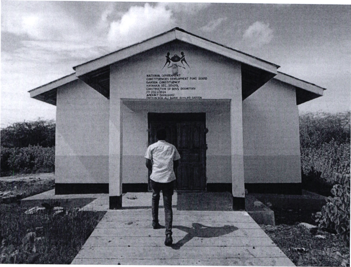
Hashaka Secondary School-Construction of Boys Dormitory
