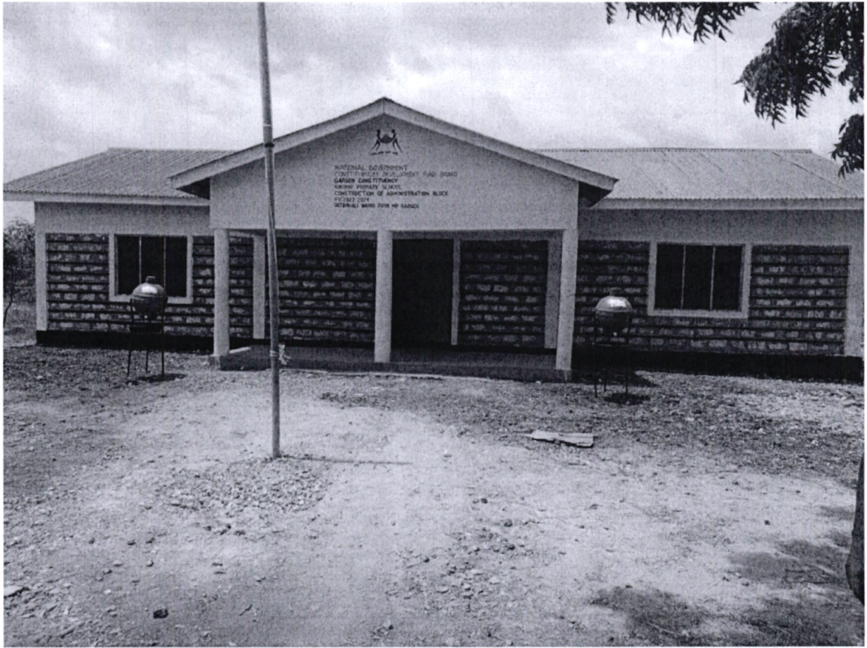
Kikomo Primary school – Construction of an Administration Block.
