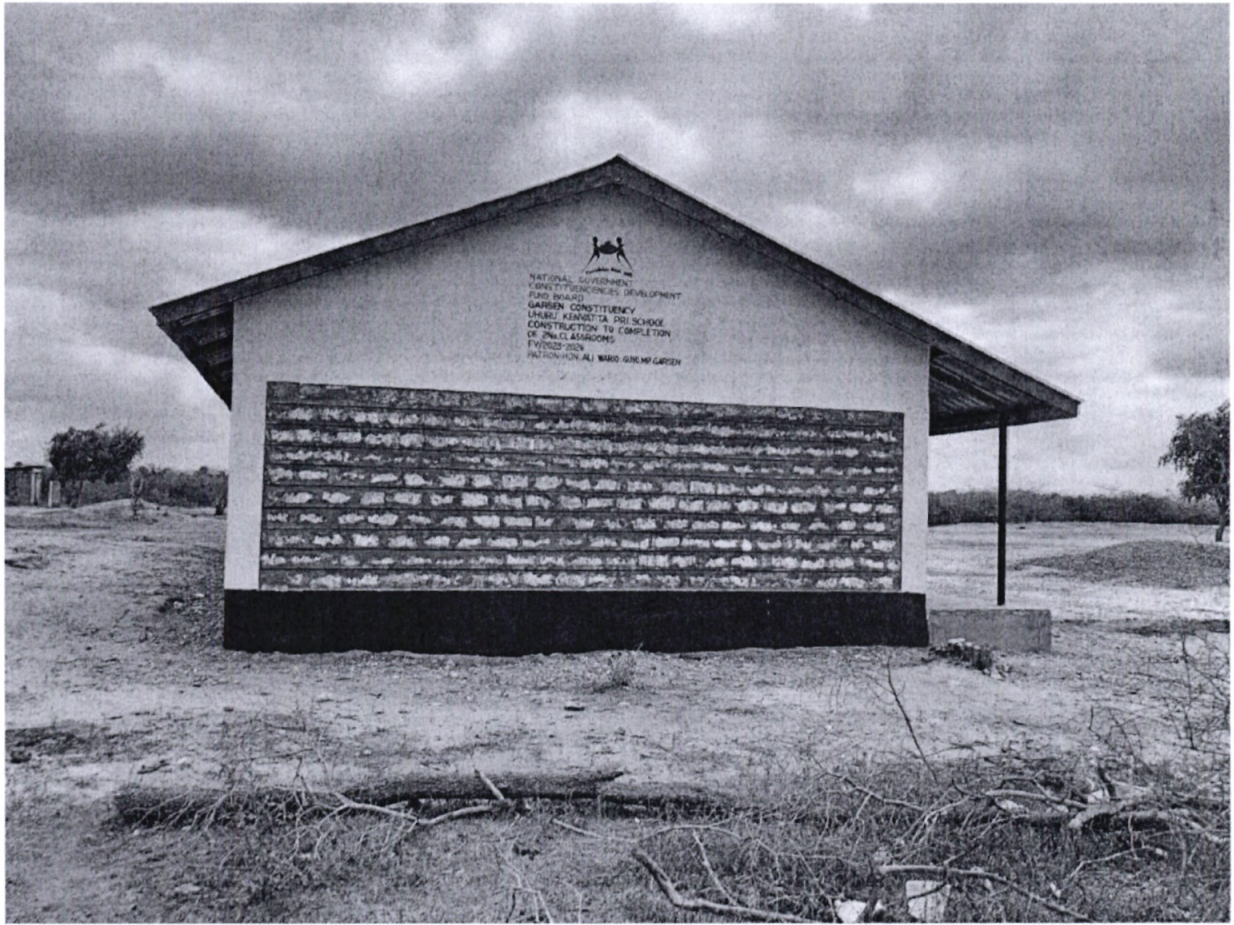
Uhuru Kenyatta Primary school – Construction of 2No. of classrooms
