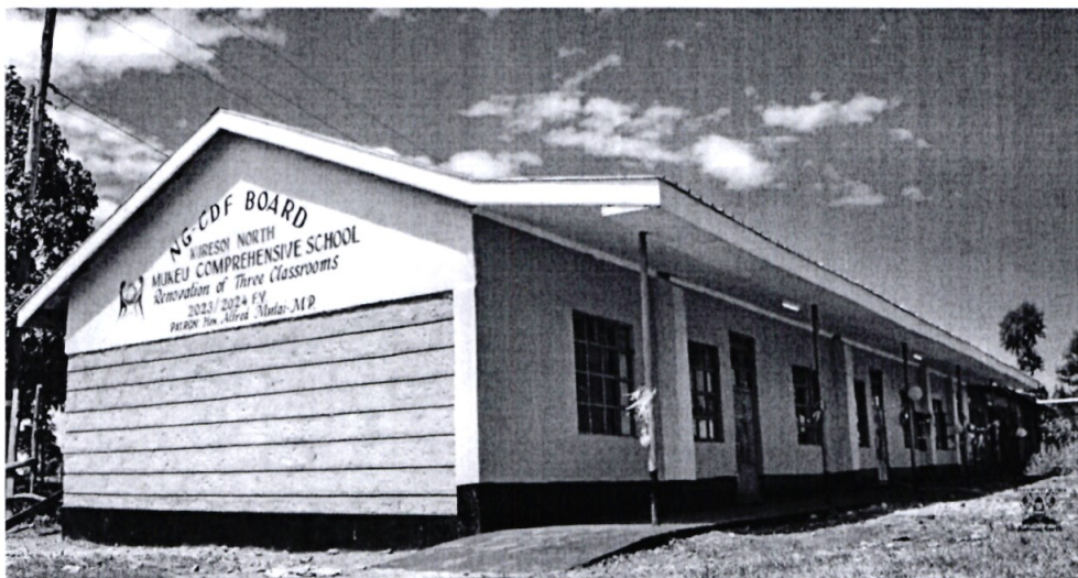
Mukeu Primary School-Renovation of classrooms
