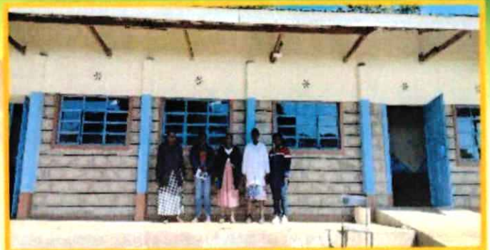
Construction of a classroom & Administrative Office at Kaptelo Girls in Bungoma County
