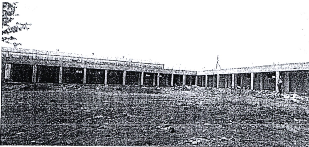
Imara secondary school under construction.
