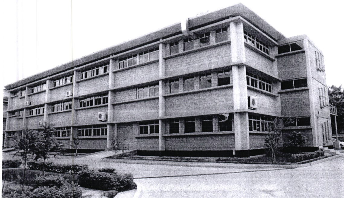
Energy resources technology laboratory and demonstration block at KIRDI KISUMU
