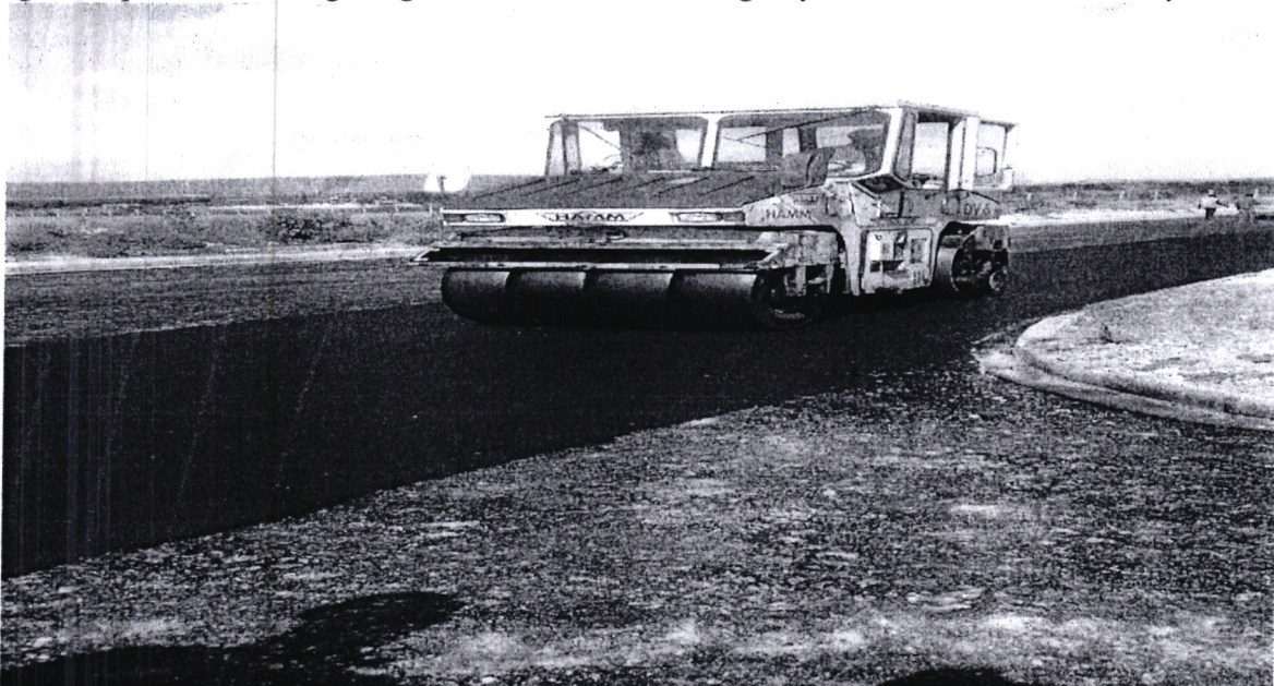
Road networks been built at EPZA
