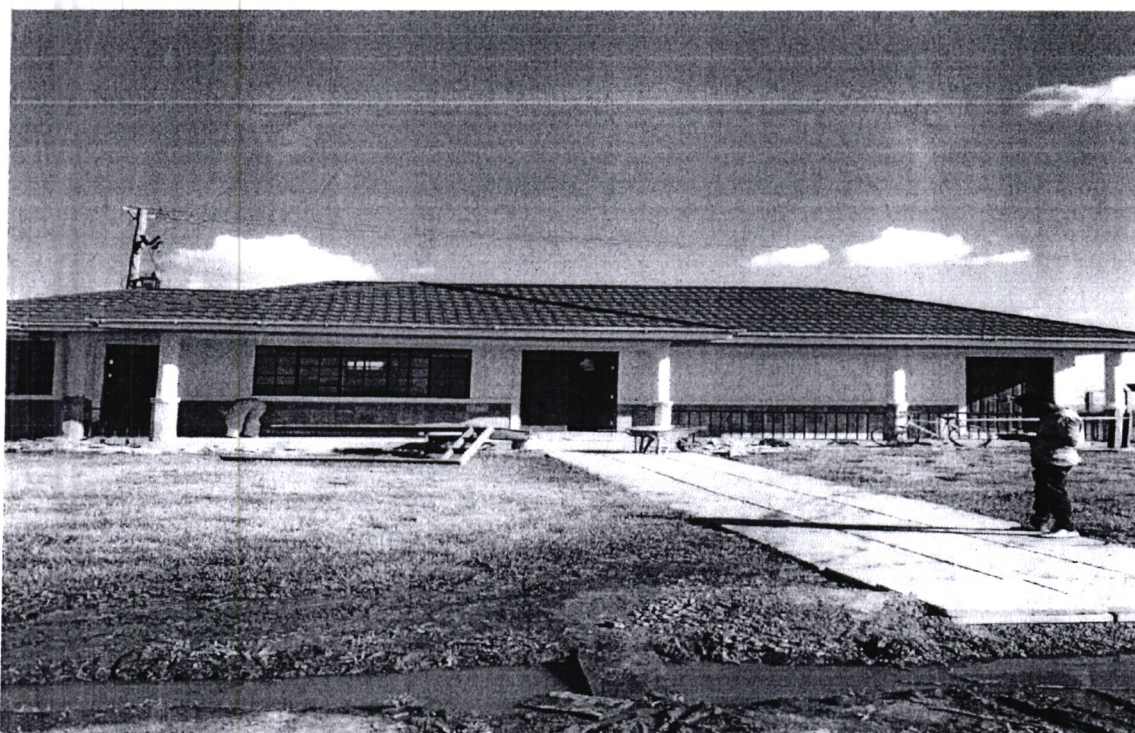
Front view of completed proposed Administration office of the site
