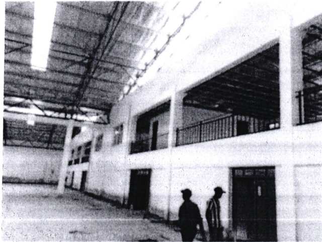
Internal view of the cluster, (Mezzanine) Railing and steel doors in place
