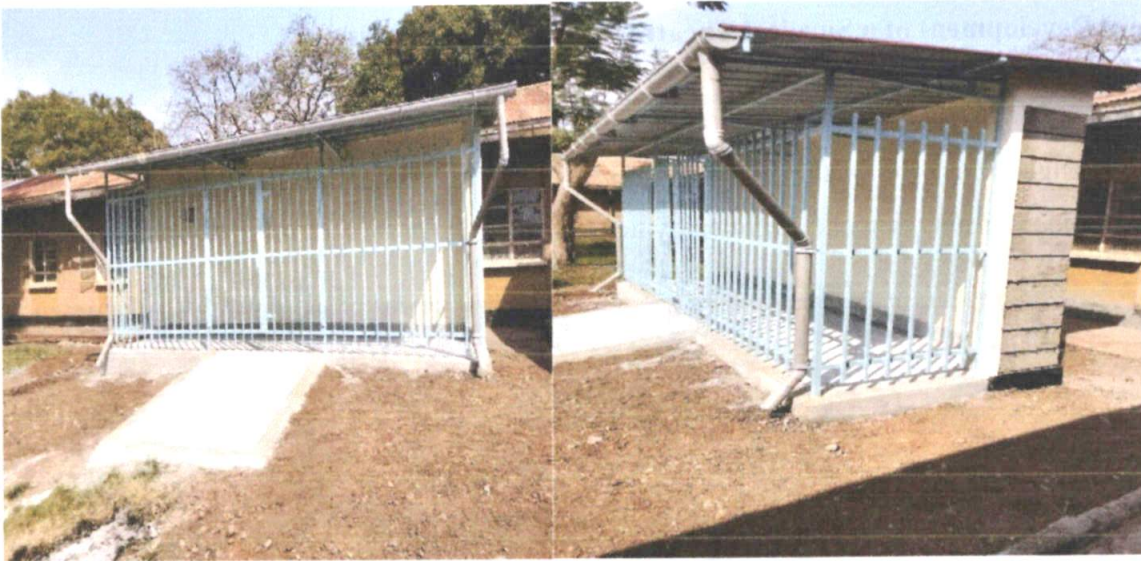
Oxygen rack plant
