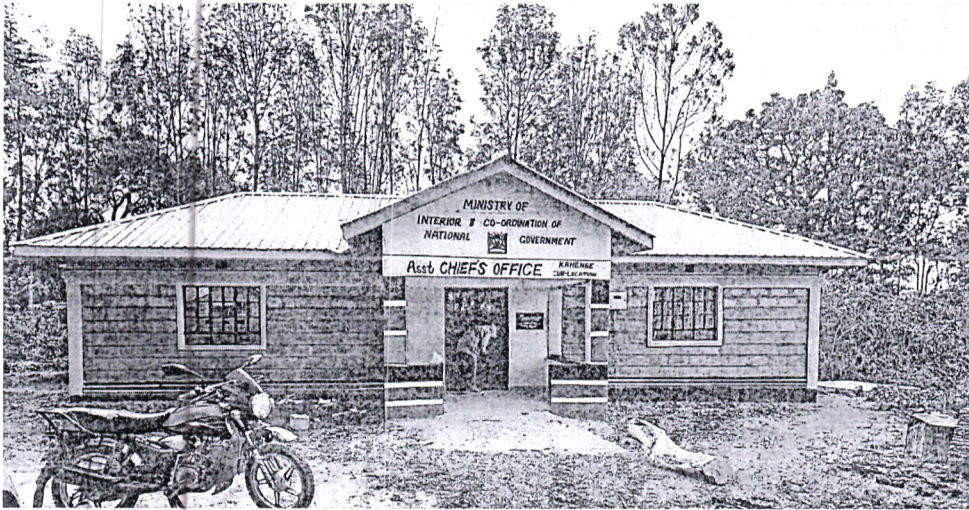
Construction of Kahembe assistant chief's office
