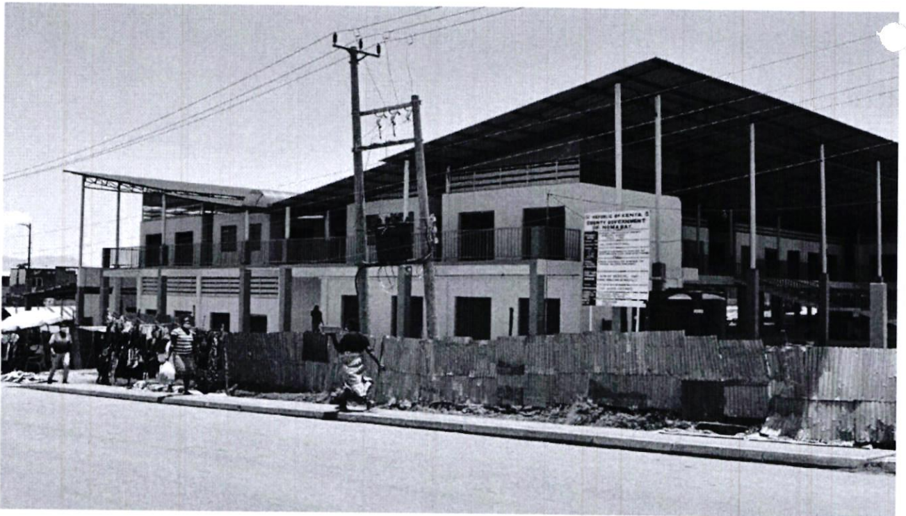
Image 3: Ongoing Construction of Homabay Municipal Modern Market
