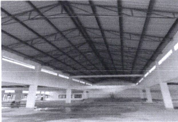
ON-GOING CONSTRUCTION OF 1500 CAPACITY DINING HALL AT CHWELE GIRLS HIGH SCHOOL
