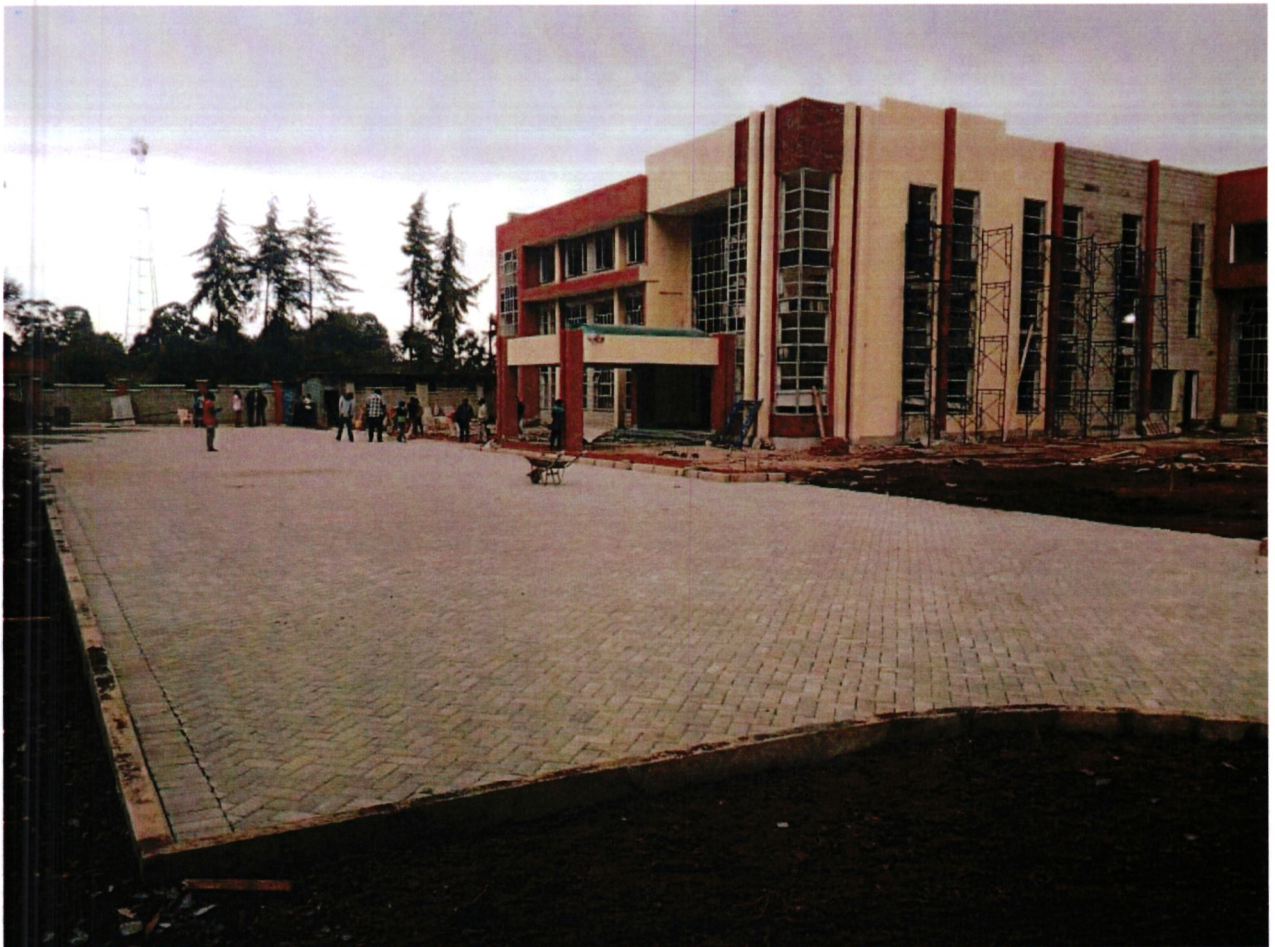
ELDORET REGIONAL OFFICES WORK IN PROGRESS
