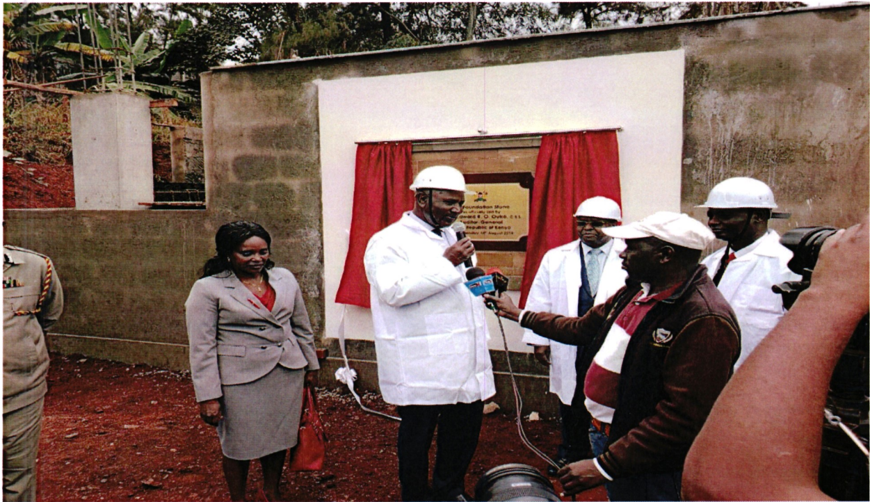
EMBU REGIONAL OFFICES UNDER CONSTRUCTION
