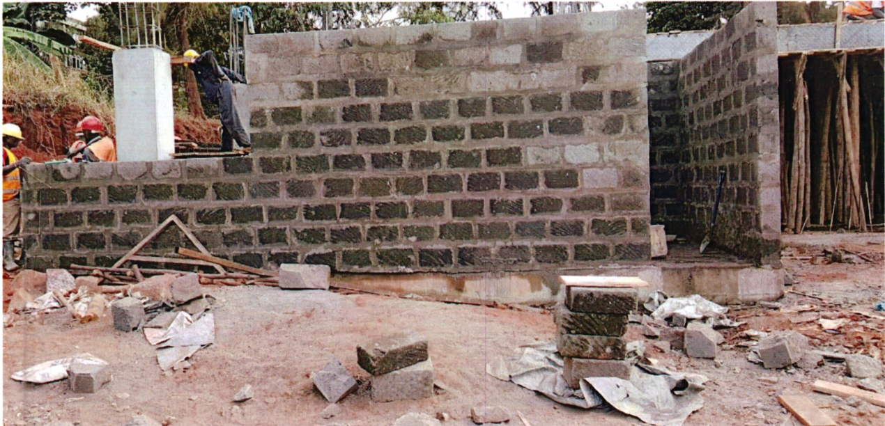
EMBU REGIONAL OFFICES UNDER CONSTRUCTION
