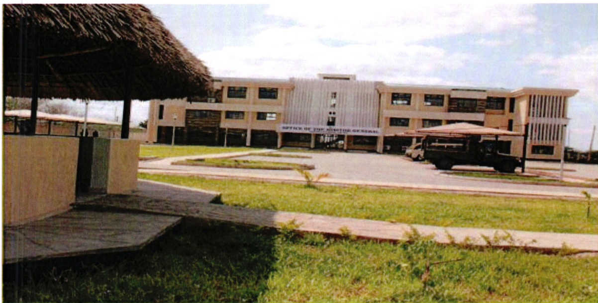
COMPLETED GARISSA REGIONAL OFFICES
