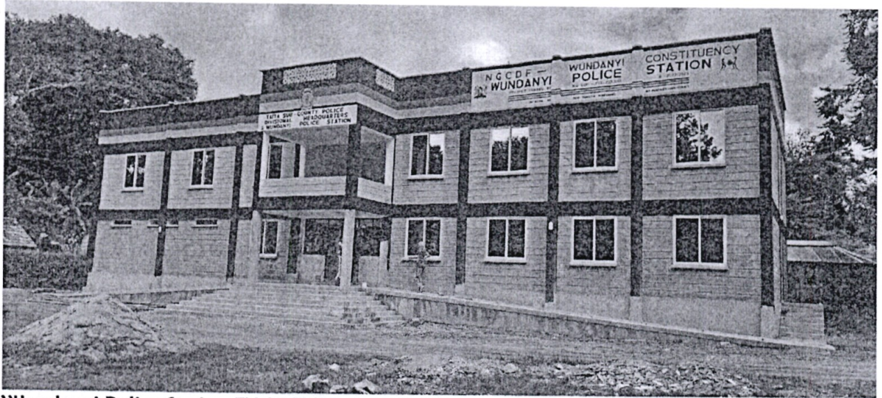
Wundanyi Police Station FY 2021/22 & 2022/23: Construction to completion of a new modern police station.
