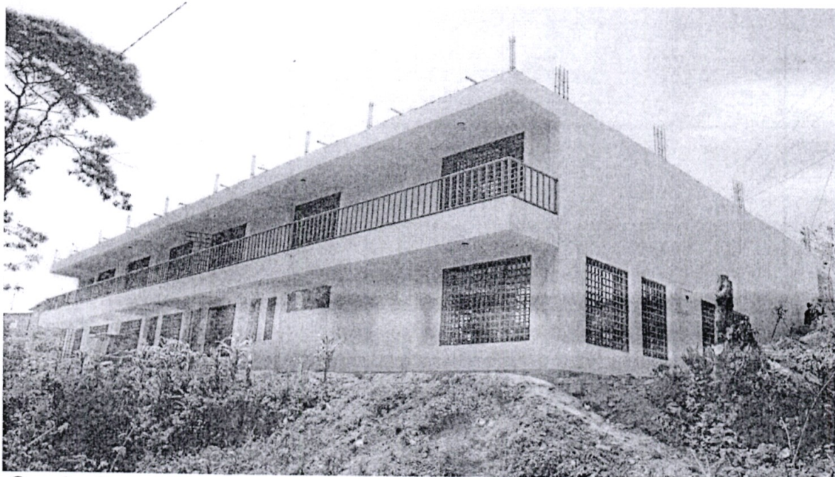
Ongoing Project-Wundanyi ACC Administration Complex FY 2020/21 & 2021/2022
