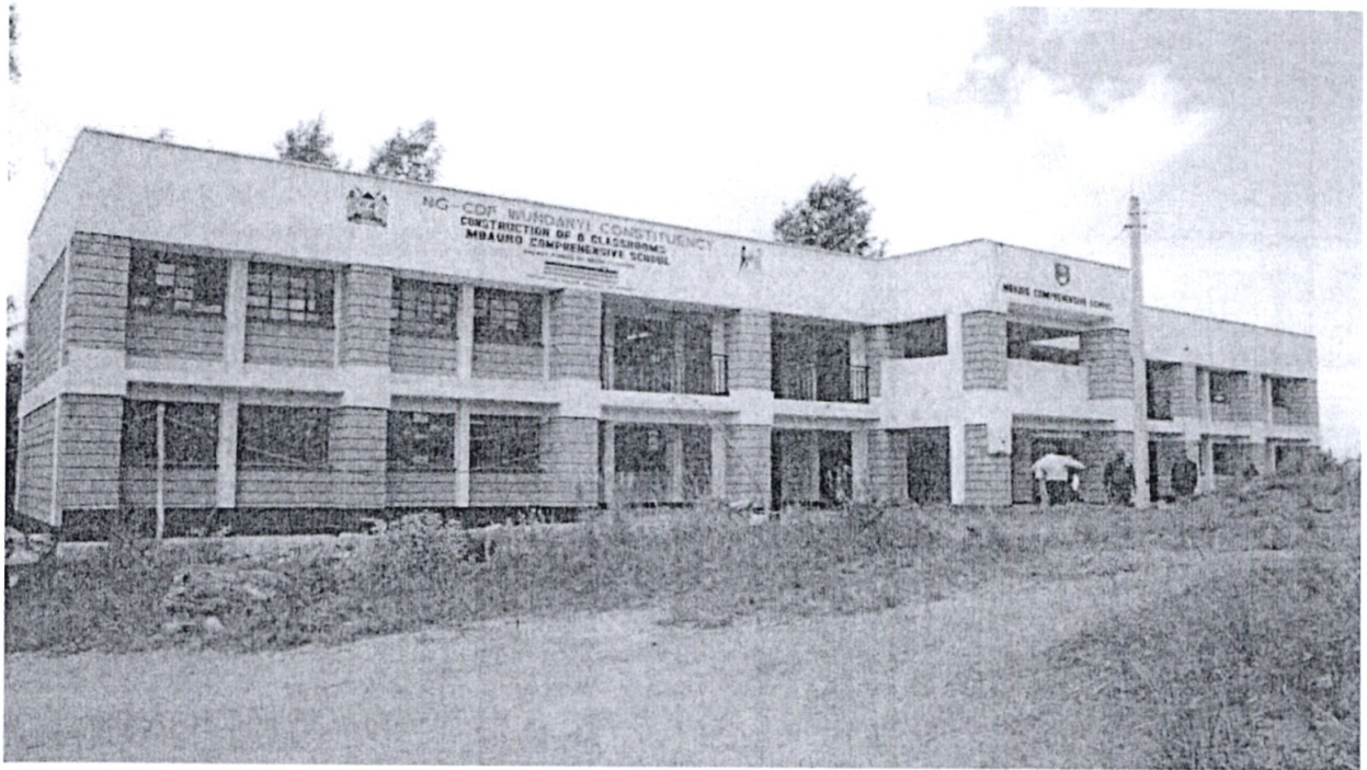
Mbauro Primary School FY 2022/23 & 2023/24-Construction to completion of 8 storey classrooms
