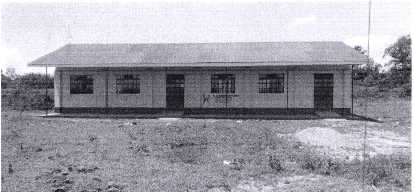
Figure 1: Mukemo Primary school. -Finished two classrooms
