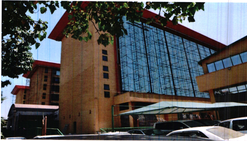
The New Mitihani House (Ongoing Project)
