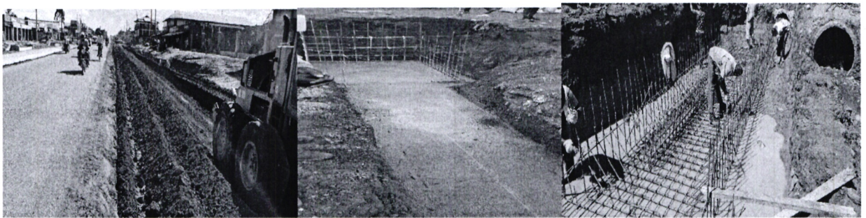
Figure: Upgrading Kanduyi sangalo to a dual road 40% complete.
