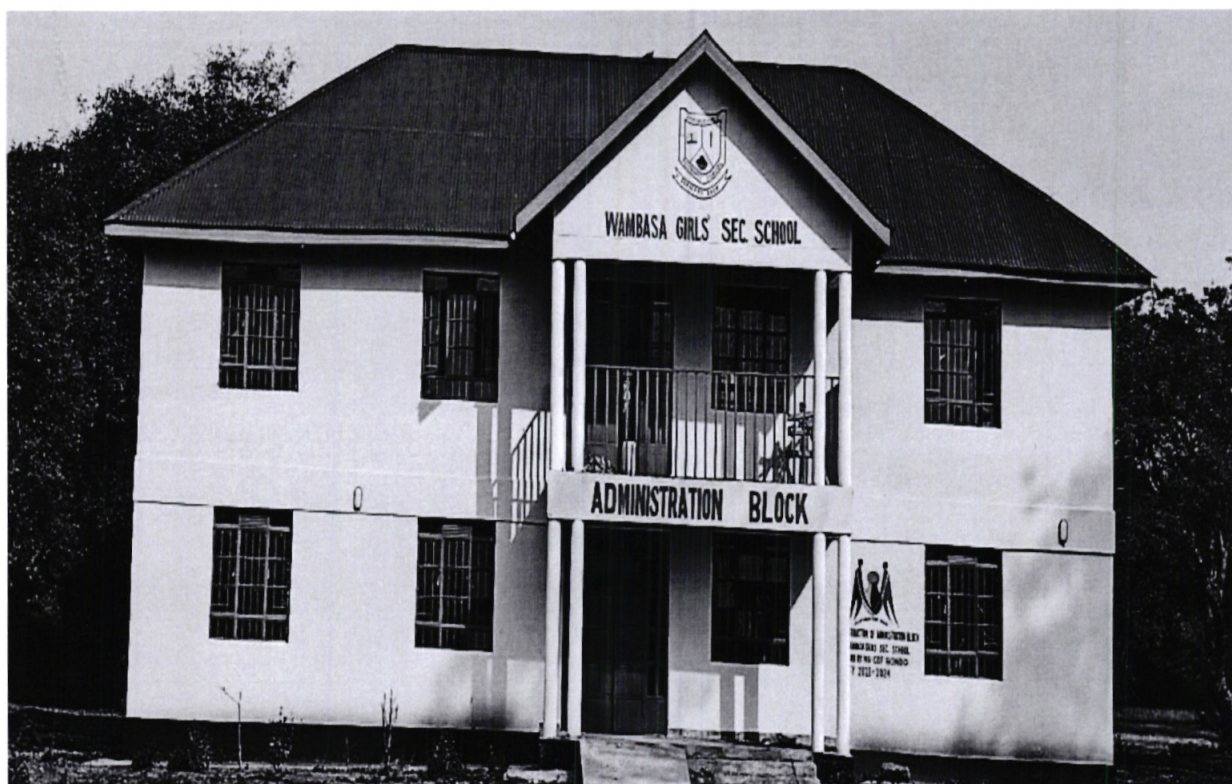
Construction of Administration block at Wambasa Girls secondary
