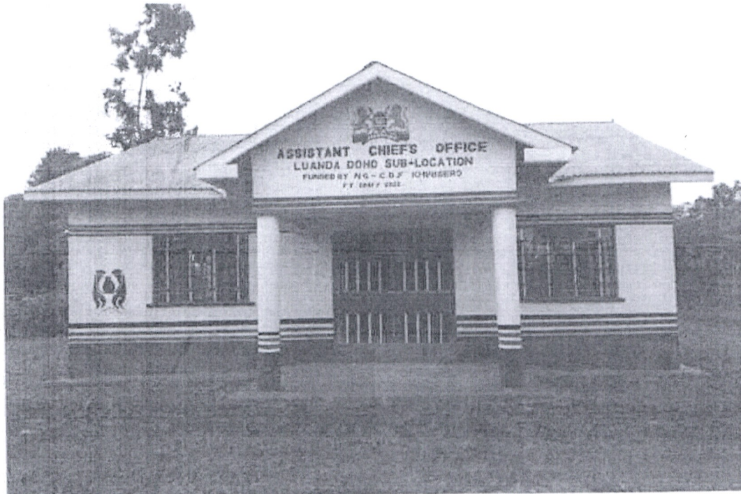
Assistant Chief's office, Doho Sub-Location - Complete, handed over and in use.
