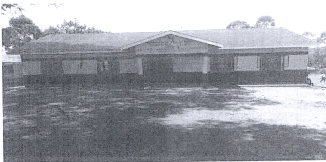
Mwibelenya Primary School - Construction of a modern Administration Block. Complete, handed over and in use.
