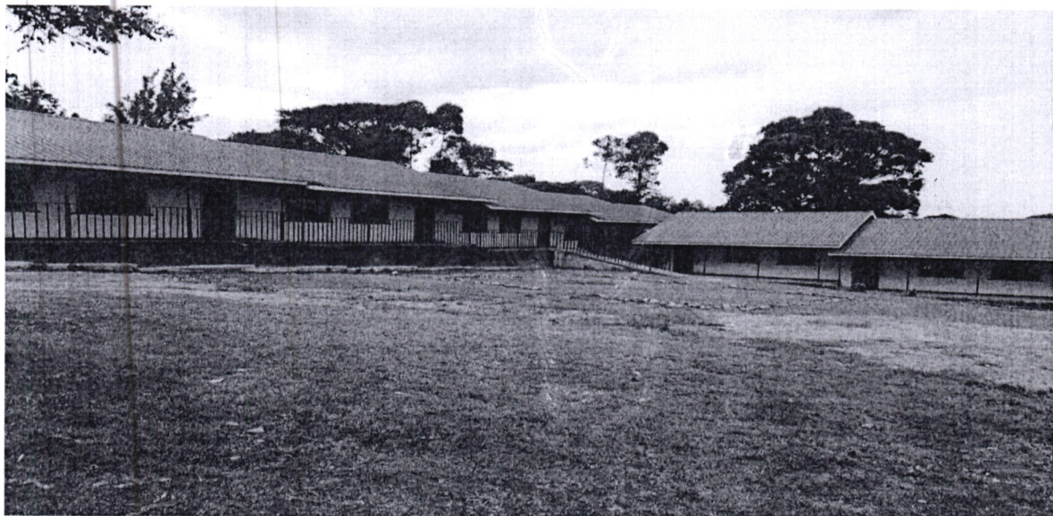
SHILONGO PRIMARY SCHOOL EIGHT NUMBER CLASSROOMS
