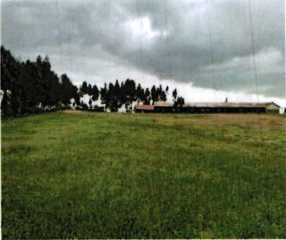
Completed Levelling of school playground at Enabelbel Primary school
