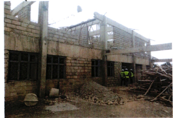
Ongoing construction of Nyabondo Trauma Centre along Kisii – Abero road.
