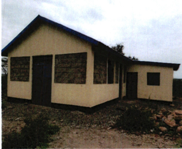
Construction of Kalobeiyei youth center along Lokitaung - Kalobeiyei road
