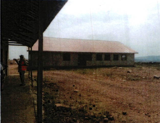
Ongoing Construction of Goanyinyo Primary School
