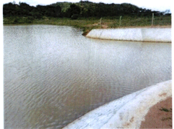
Construction of an earth dam at km 86 between Kibwezi - Kitui road
