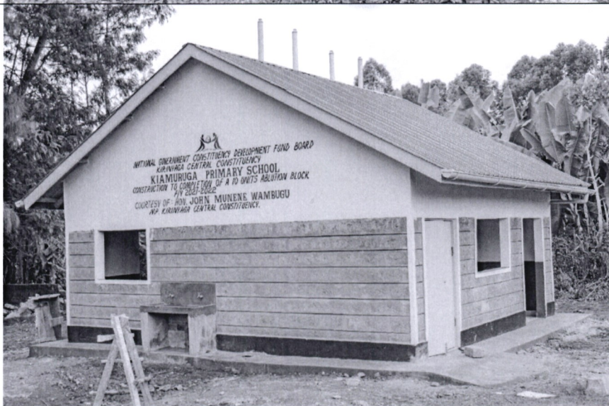
Pupils Ablution Block constructed to completion at Kiamuruga Primary school.
