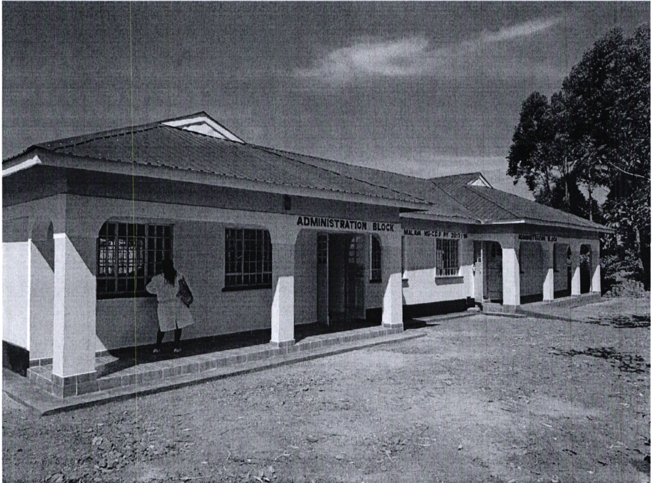
Namagara Secondary School construction of Administration Block funded by Malava NGCDF Financial Year 2018/2019
