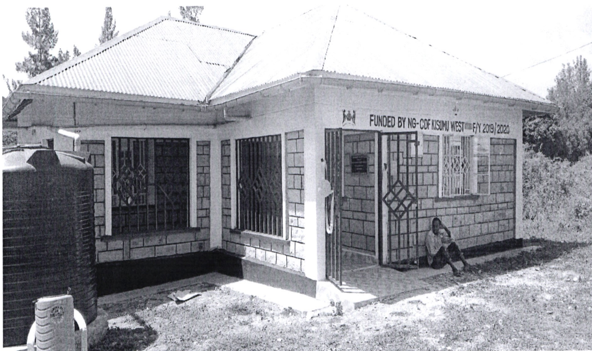
Construction of Assistant Chief Office –south Kapounja funded 2019/20, implemented 2021/22
