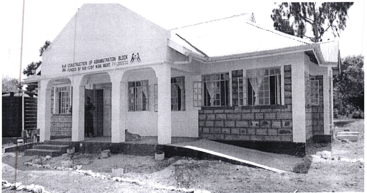
Construction of administration block at Oyiengo Primary
