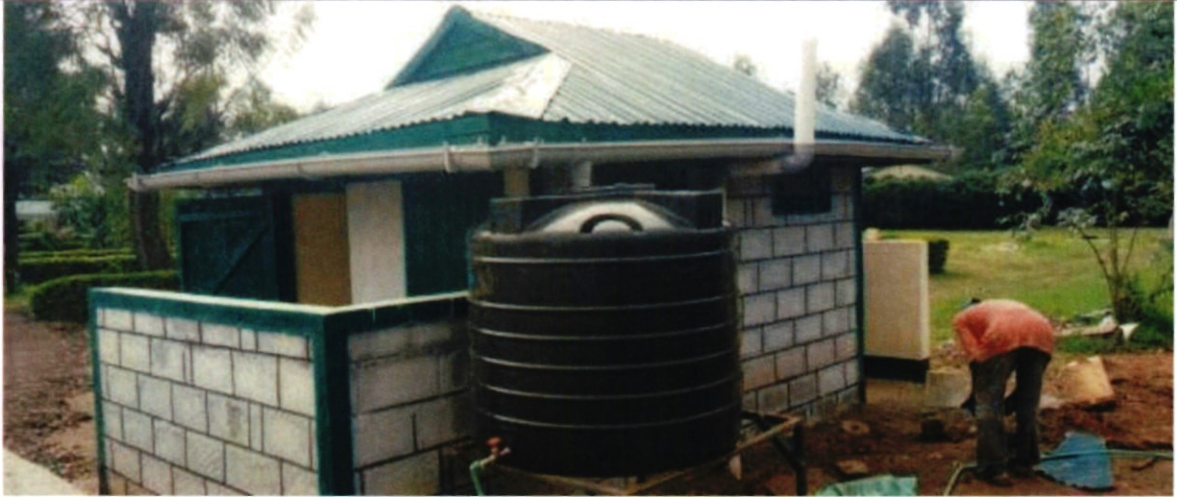
A sanitation Facility Constructed by KURA for Itando Vocational College for the deaf in Vihiga County.
