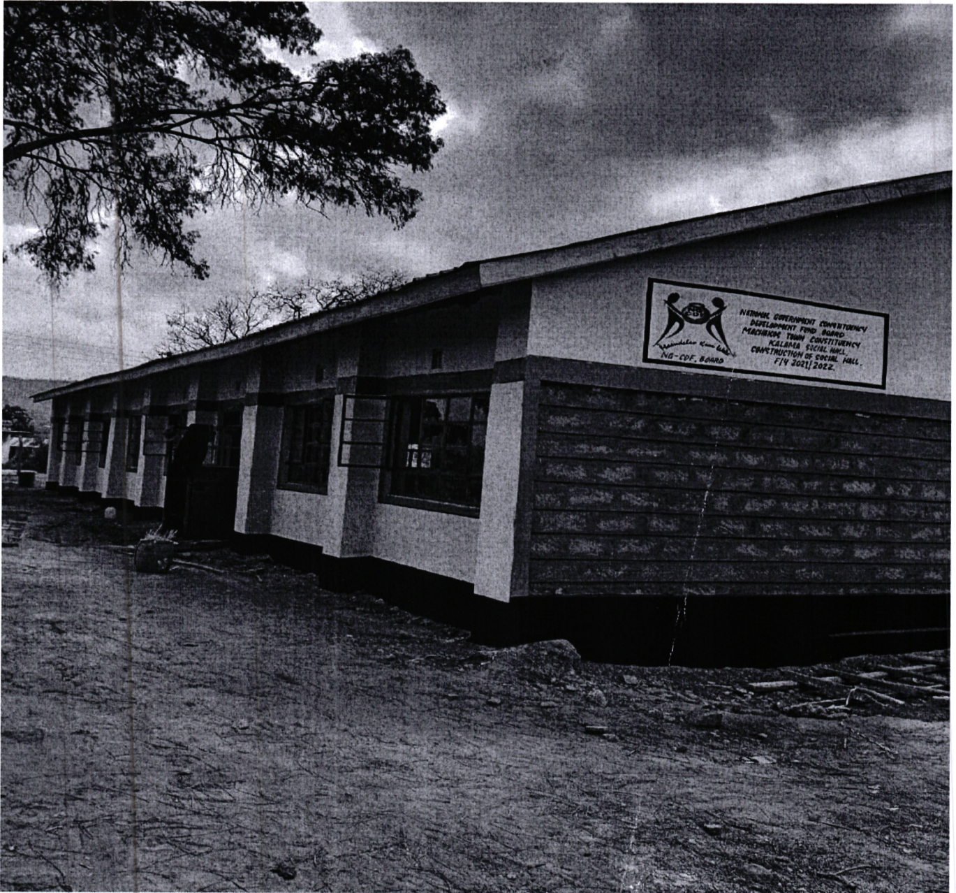
Construction of Kalama social hall – Ksh 2,000,000
