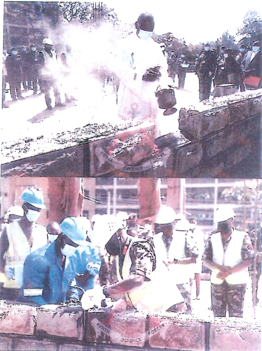
Chief of Defence Forces Laying Foundation of New Anglican Church at Defence Headquarters
