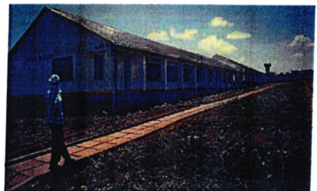
New KMTCC Admin and Classroom Block at ICRH
