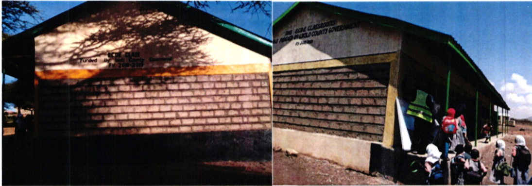
ECDE Classrooms in Merti Sub County
