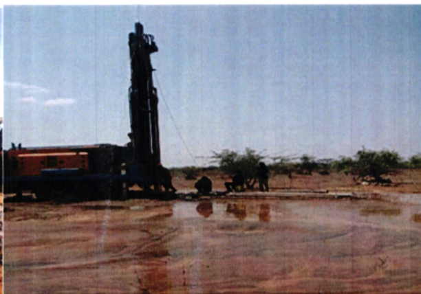
Drilled Borehole in Cherab Ward
