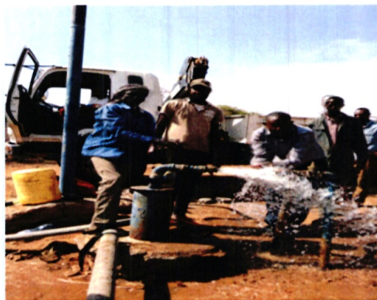
Borehole Drilled in Belgesh
