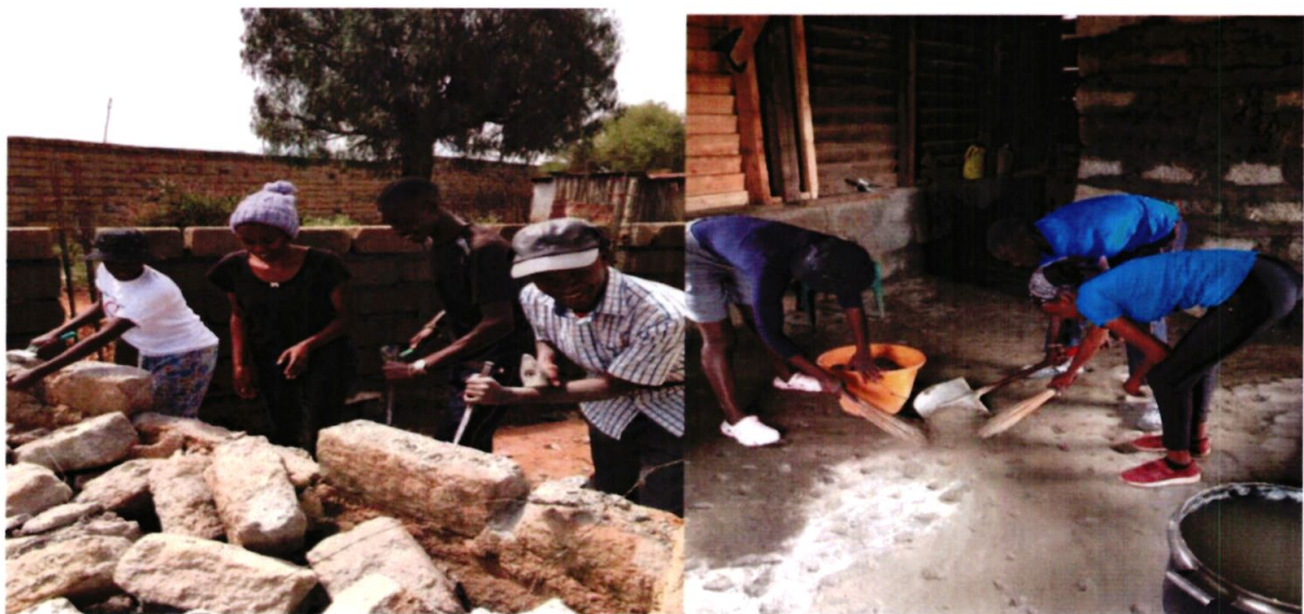
Award participants from Laikipia and Egerton Universities at Gilgil Highway Primary School during a Gold Residential Project undertook to partition the kitchen with a 9-course stone wall and cement the kitchen floor. Aside from that, the team repaired the kitchen's brick cookers and reinstalled the kitchen chimneys
