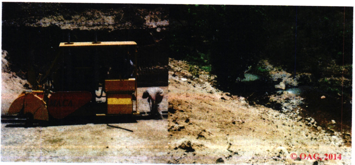
Picture 4: Quarrying Activity in Mitunguu, Meru
