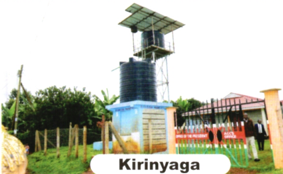
Solar powered water supply from Kiburu borehole in Ndia Sub County
