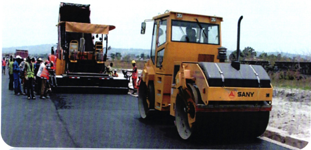
Figure 6: Road Maintenance Project in Progress
