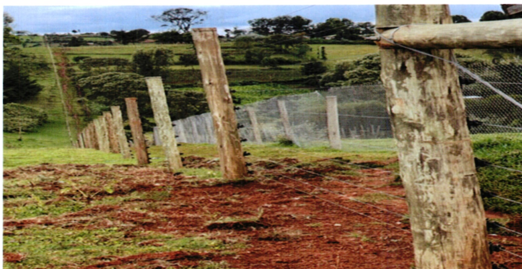
Picture 1: Erected Boundary Fence Along Maasai Mau
