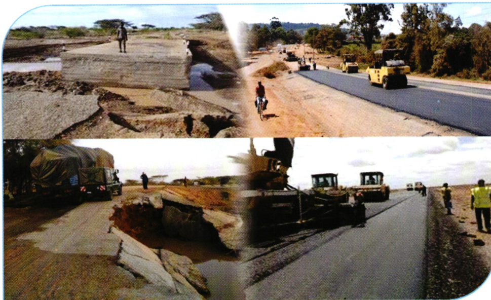
Figure 21: Rehabilitation of key infrastructure
