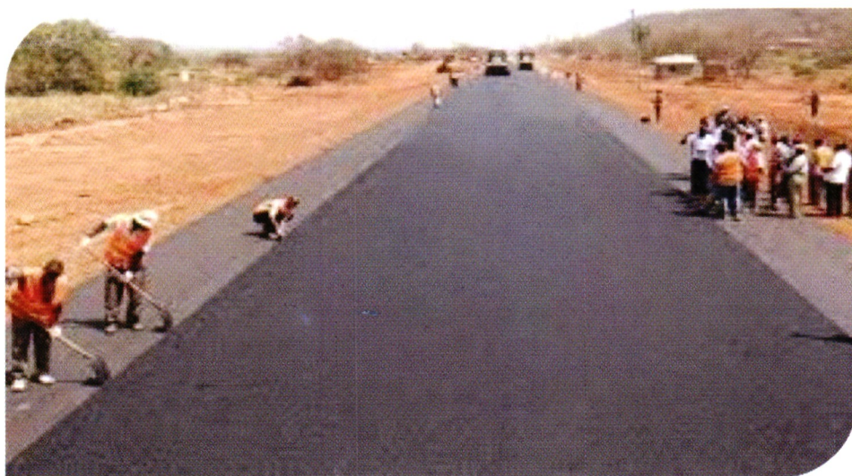
Figure 22: Construction of the Kibwezi- Mutomo- Kitui Highway
