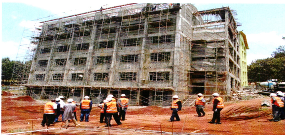
Figure 16: Construction of Tuition Block Phase II at MUT
