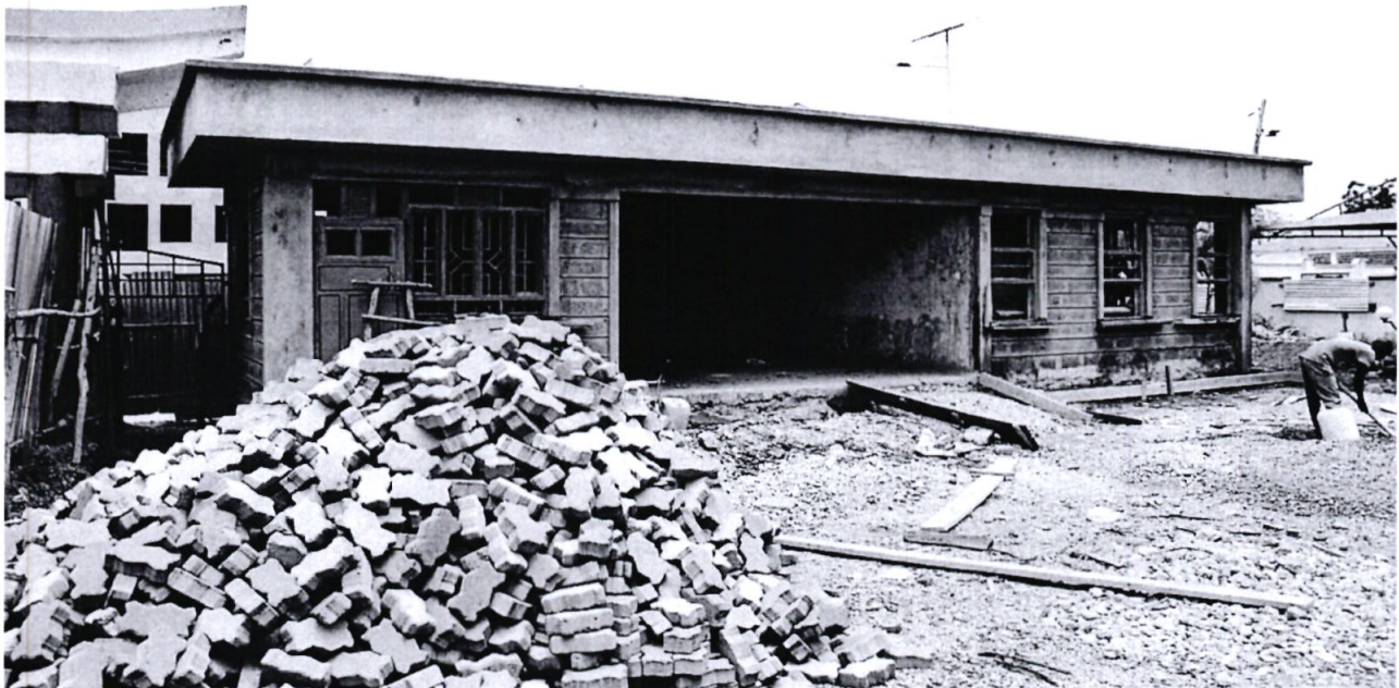
Picture 12: Construction of Visitor's Waiting Bay
