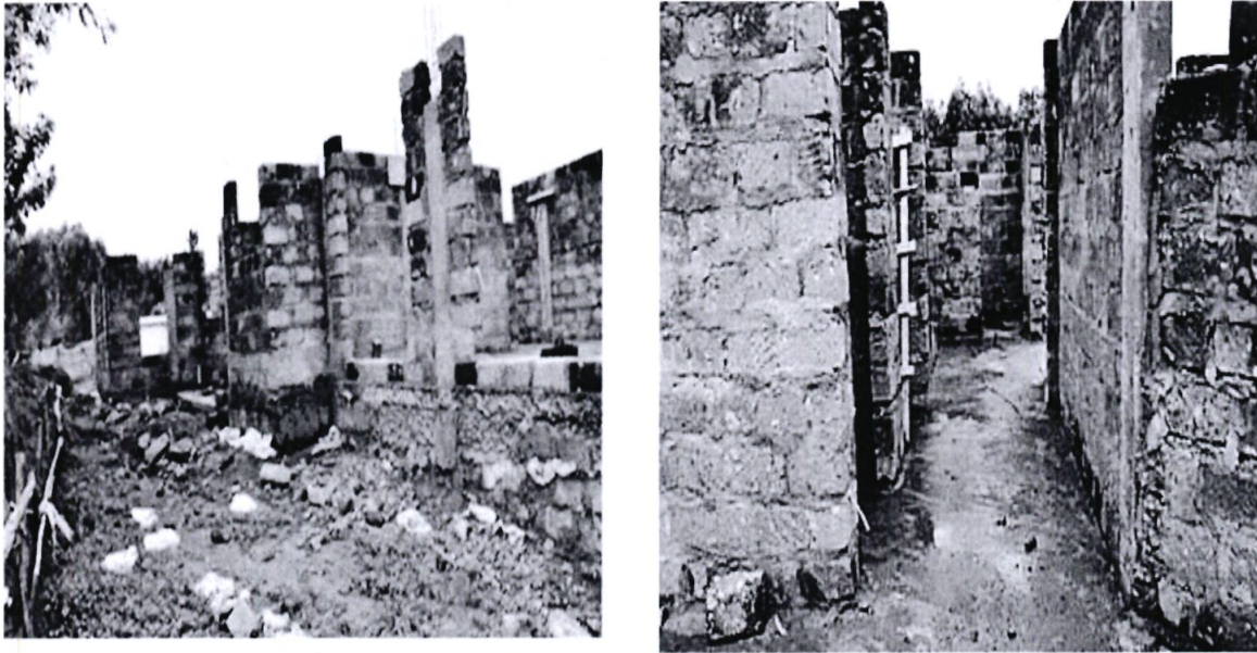
Picture 11: Construction of Speaker's Residence
