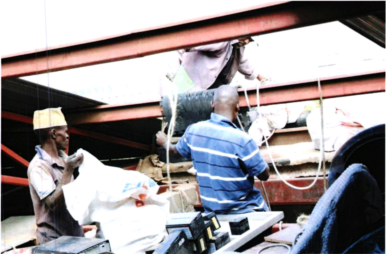
Workers commencing construction works at the Commission House in November, 2020
