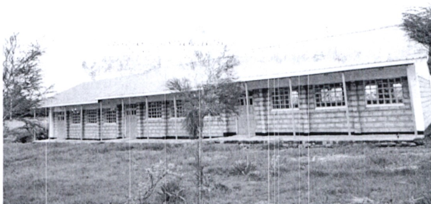
Ndoroto primary school: Construction of 3 classrooms and purchase of 120 desks
