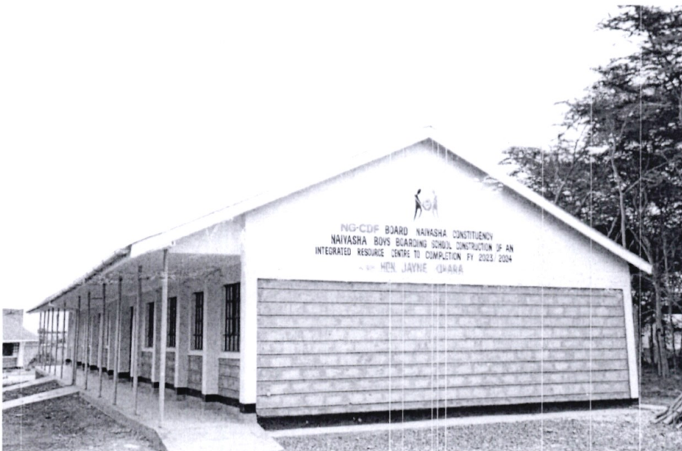
NAIVASHA BOYS BOARDING PRIMARY SCHOOL: ACTIVITY; Construction to completion of an integrated Learning Resources Centre
