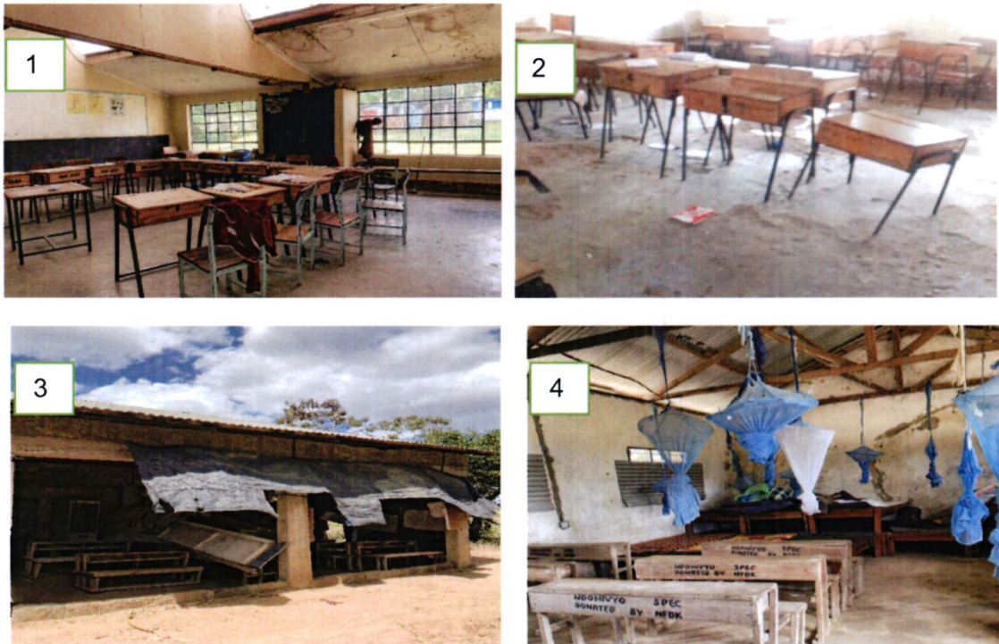
(1) Maseno School for the Deaf classroom with a damaged board and ceiling, (2) SA Thika School for the Physically Handicapped had potholes in classrooms, (3) An incomplete classroom in use at Ndohivyo Special School for the Mentally Handicapped and (4) Ndohivyo Special School for the Mentally Handicapped using the same room as a classroom, and a dormitory
