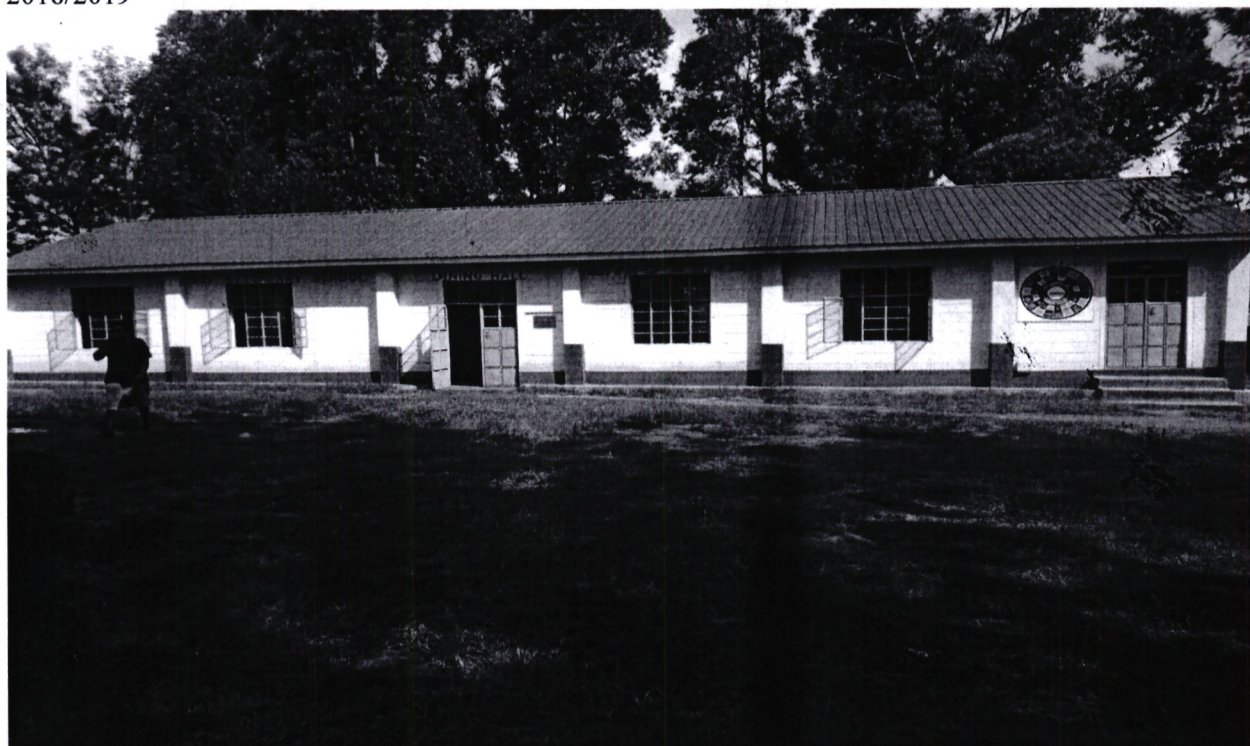
Figure 4. Soy Secondary School completion of Dining Hall in the financial year 2018/2019 now in use.
