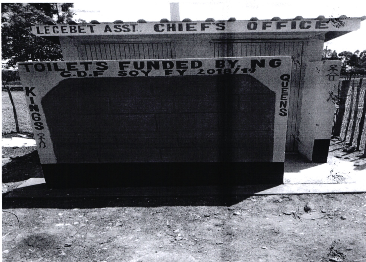
Figure 6. Legebet Assistant Chiefs Office construction of 2 door pit latrine in the financial year 2018/2019
