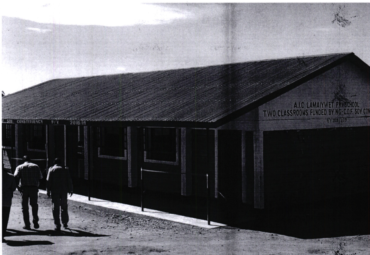
Figure 3. AIC Lamaiywet Primary School construction of Two classrooms to completion in financial year 2018/2019
