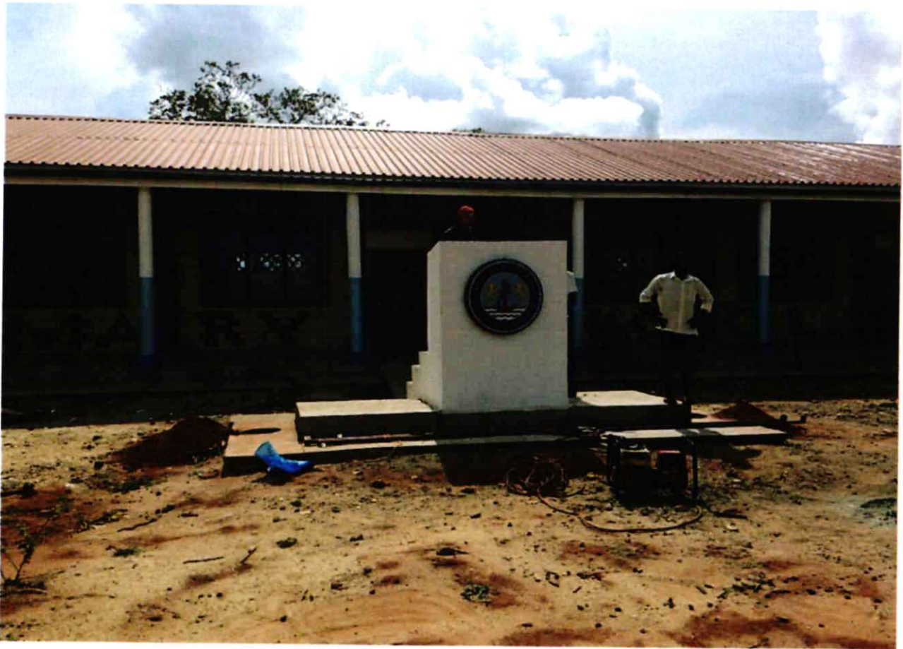
Four classrooms built by KPA at Sosodemu primary school
