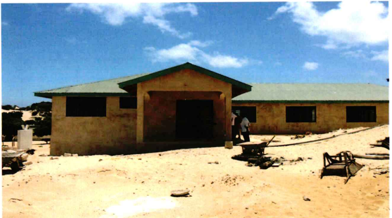
Construction of library at Bright Girls Secondary School
