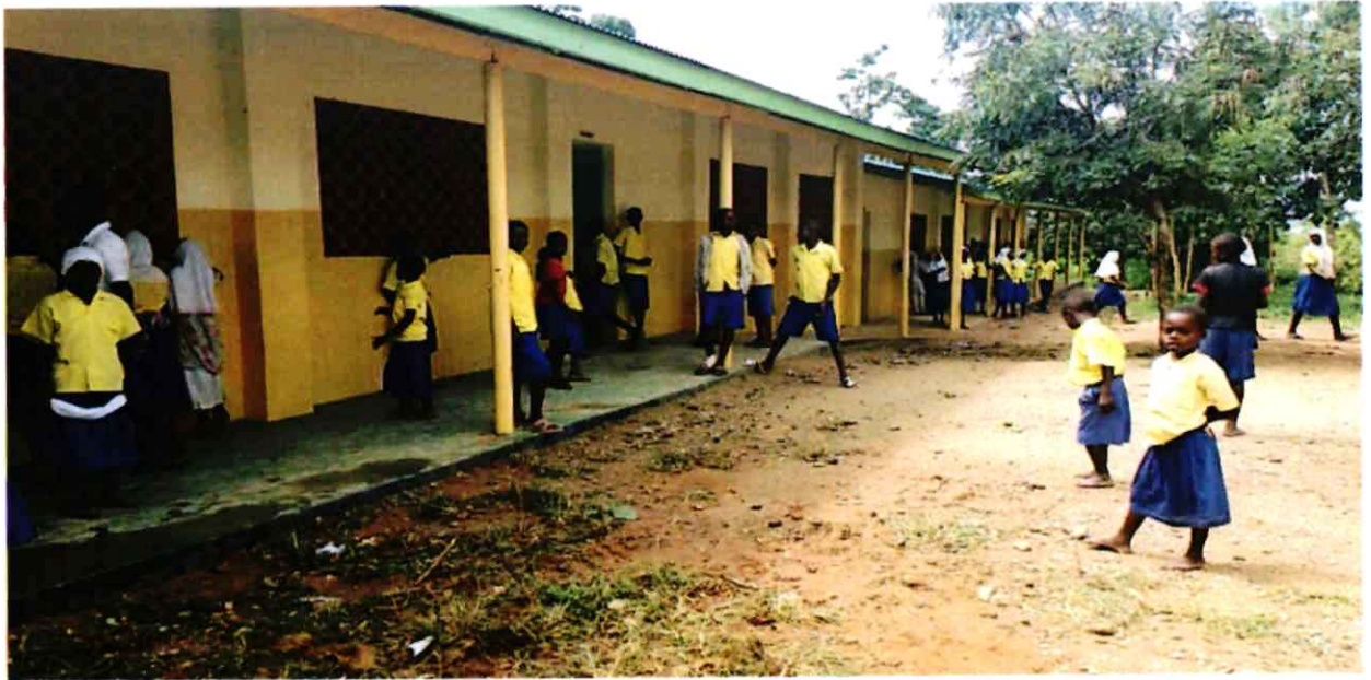
Four classrooms done by KPA at Maweu Primary School
