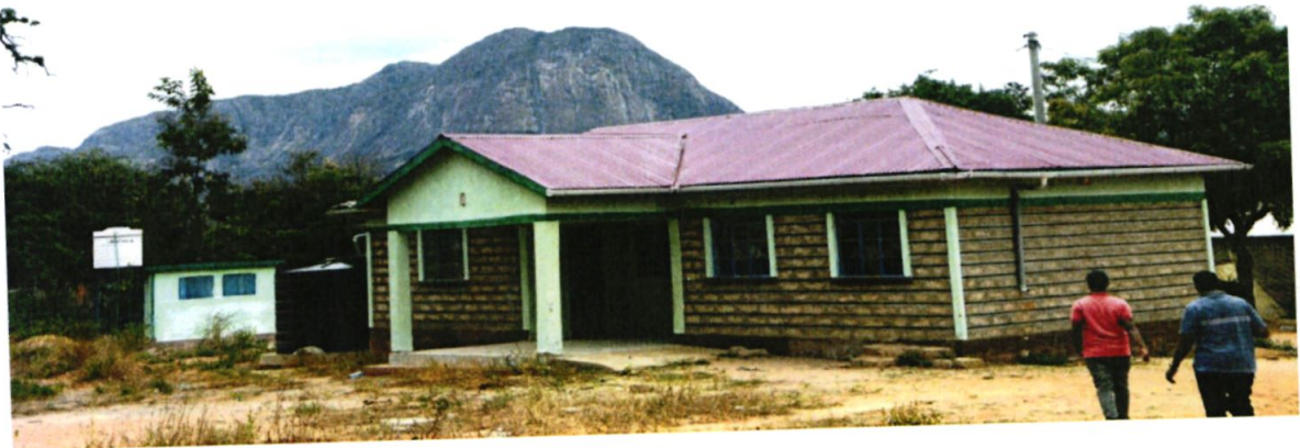
Completed Sololo ward office implemented during the financial year.
