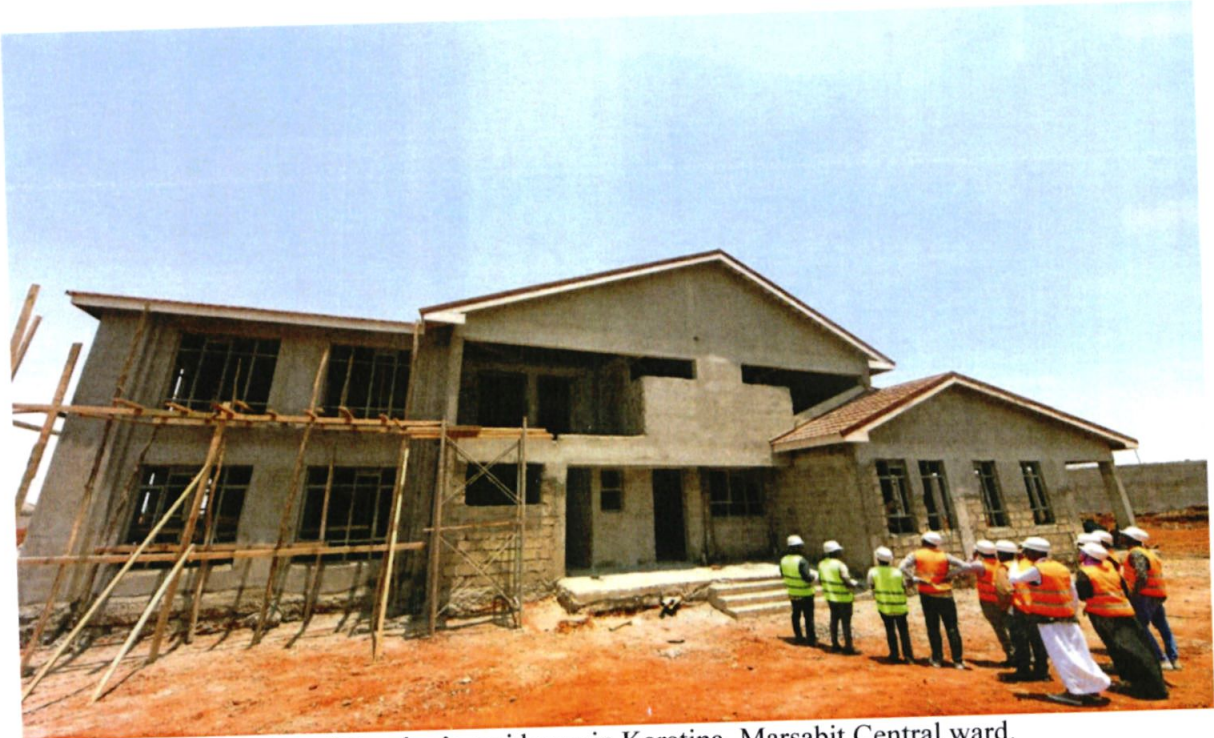
On going construction of Speaker's residence in Karatina, Marsabit Central ward.
