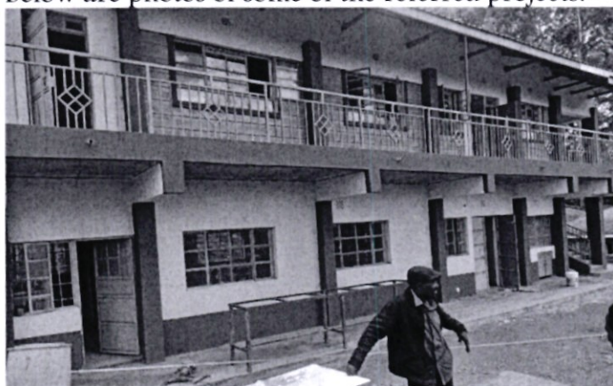
Storied laboratory completion works at Dr. Kiano Secondary School
