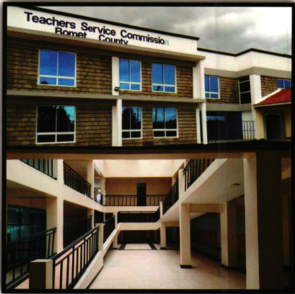
Front view of the TSC Bomet County office, constructed as some of the service improvement initiatives. The project is 95% complete.
