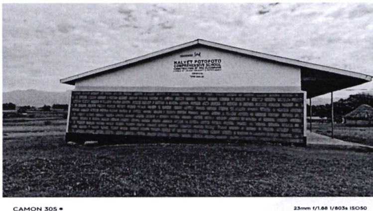
Construction of one classroom at Kalyet Potopoto Primary School.
