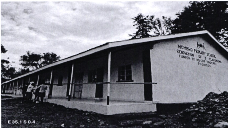
Renovation of 3 classrms at Mombwo Primary School
