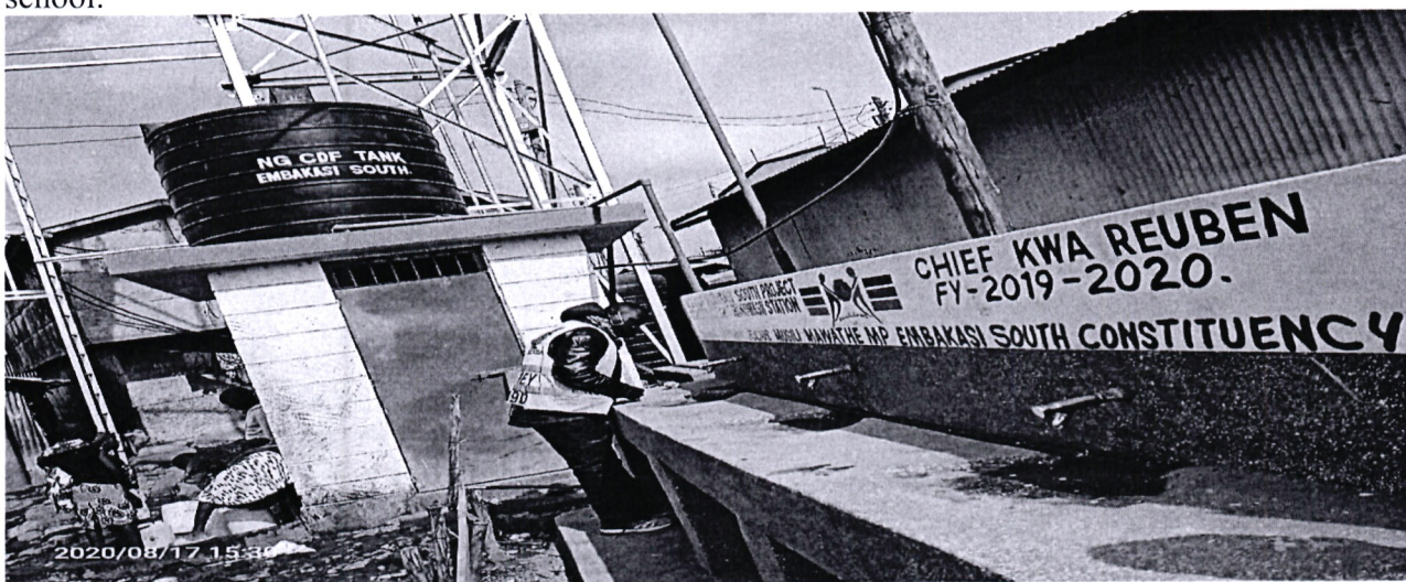
FIG 1.1 Kwa Reuben Chiefs Camp construction of Hand Washing Stations.
