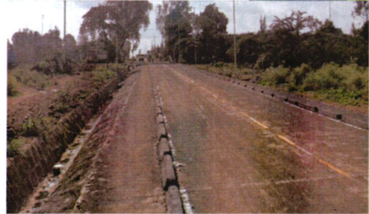
: Well aligned and stone pitched side drain along Solomon Kiguru Road.
