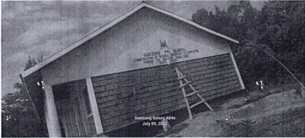
God Jope Primary -Construction of science Laboratory to completion.
