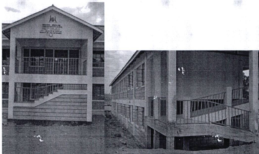
Migori Muslim Primary School (Construction of Eight classrooms to completion) which has decongested pupils learning environment.
