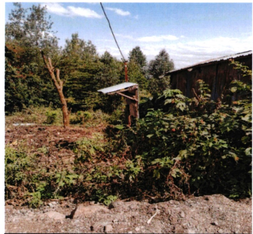
Picture 4: Service cables erected on parcels of land with non-existing households at Korompoi, in Kajiado County
