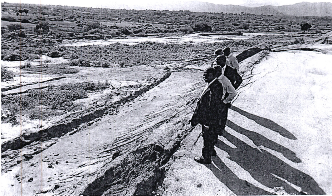
Figure 12: Area needing retention wall
