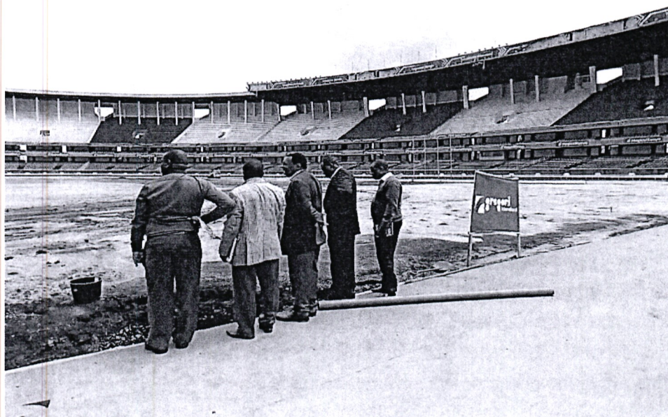
Figure 22: Ongoing refurbishment of Kasarani Main Football Pitch
