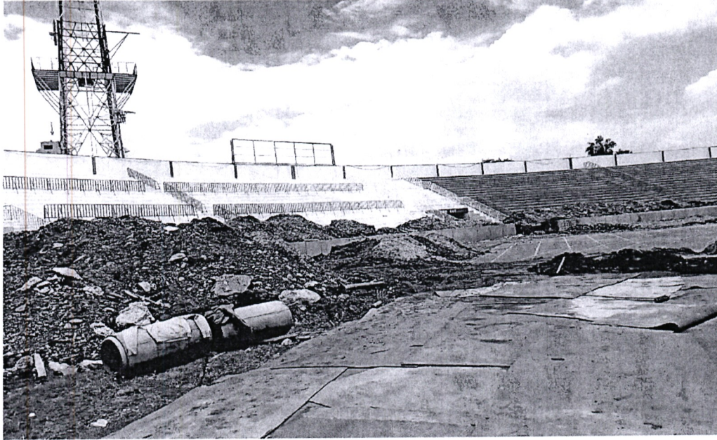
Figure 23: Ongoing Works, Nyayo Stadium
