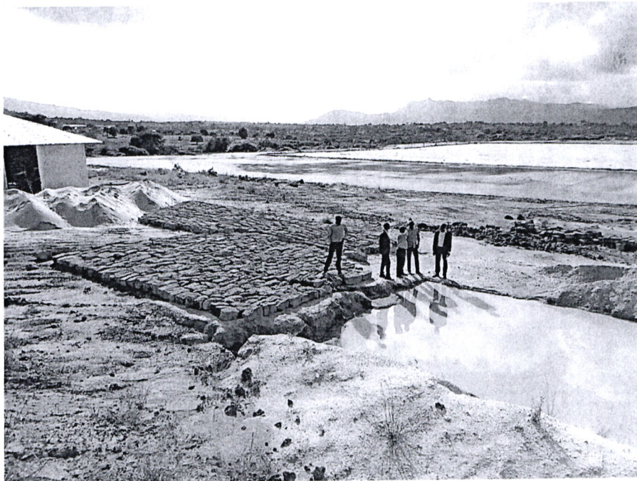
Figure 13: Underground tank excavation hampered by rain
