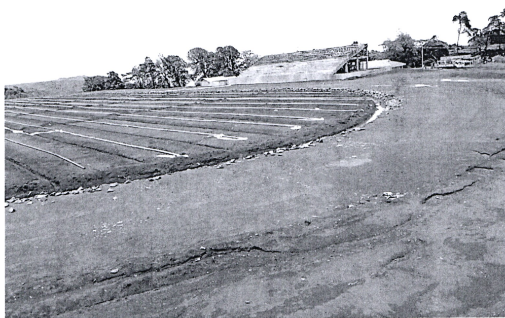
Figure 19: Ongoing works, effects of rainy weather visible
