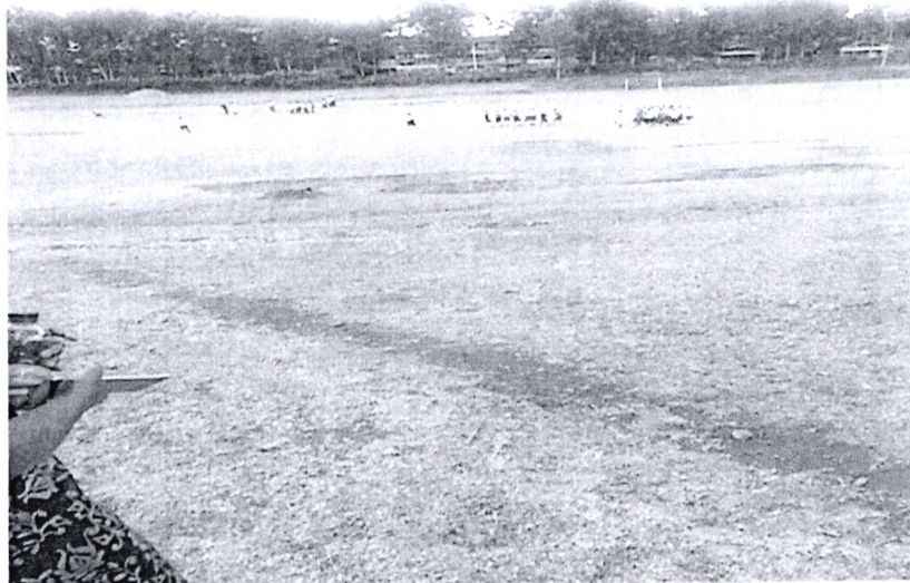
Figure 4: Karatu Stadium before the start of construction
