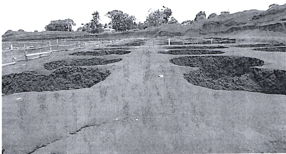
Figure 18: Foundation works, VIP Pavilion
