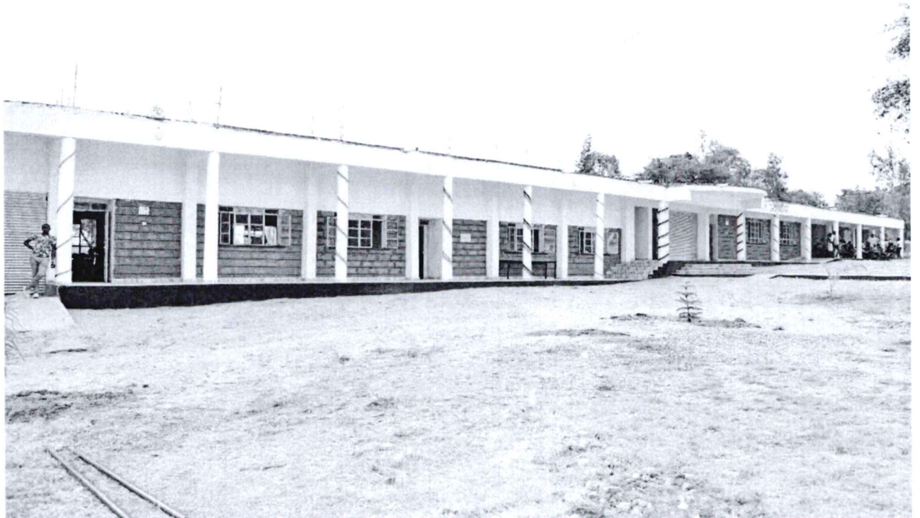
Fig. 7. Seme Teachers College; Construction of 8 Classrooms Phase I
