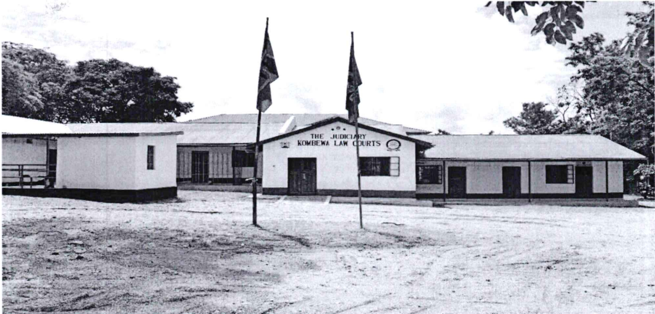
Fig. 5. Renovation of Kombewa Law Courts
