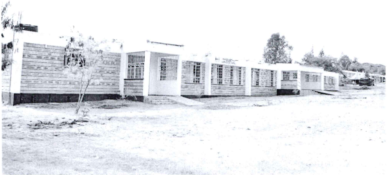
Fig. 6. Seme Teachers College; Construction of Female Hostels Phase I
