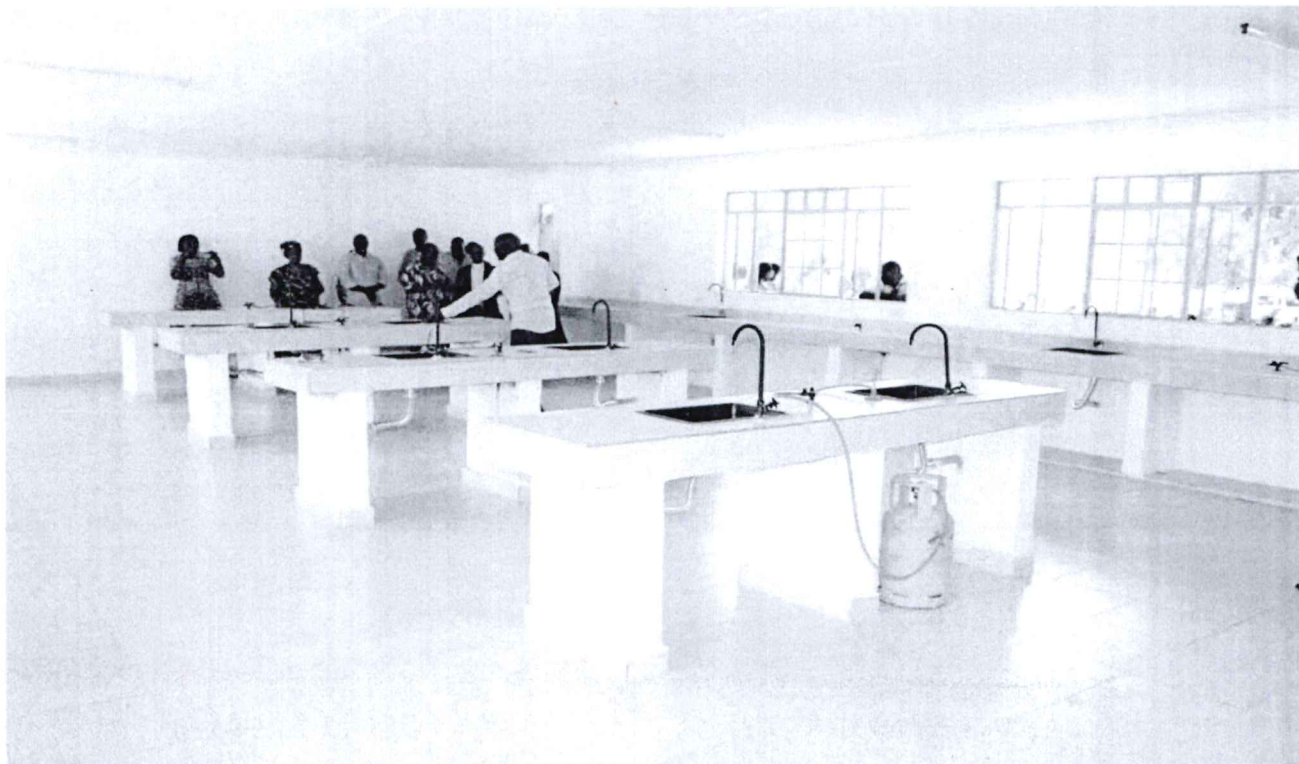
Fig. 2. Bishop Abiero Oruga Sec School; Construction of Laboratory
